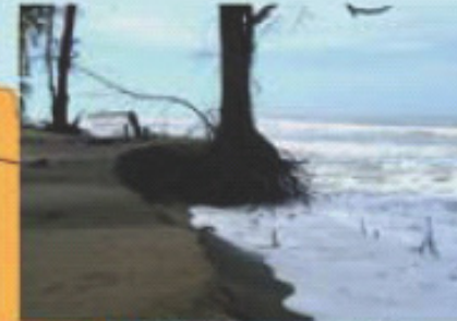
Coastal erosion and subsidence of the terrain
