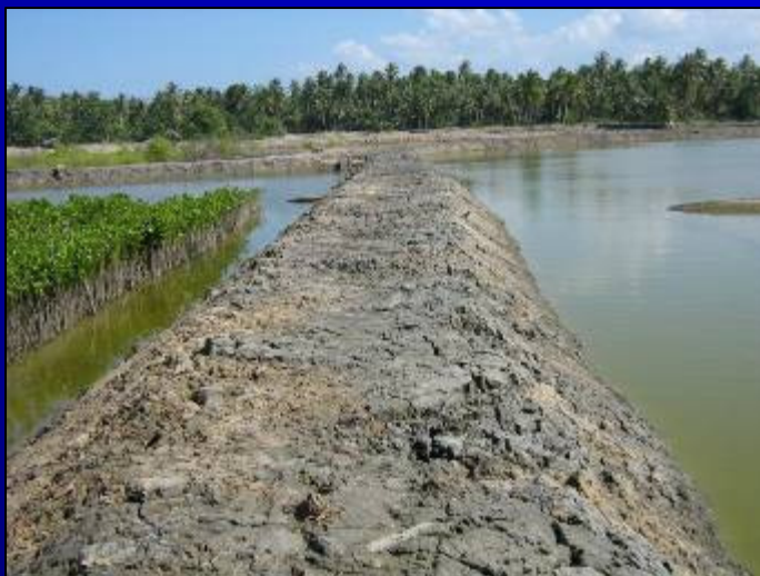
Rehabilitated pond, Banda Masen village, Lhokseumawe, showing mangrove nursery.
