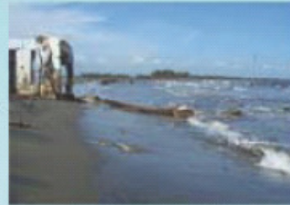
Infrastructural damage and subsidence of the terrain
